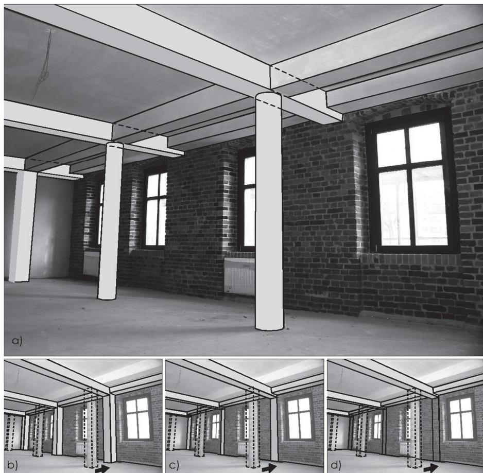
Fig. 3. The support structure of the historical wall: a) the design stage, b) the pilaster pillars, c) the visible side surface pillars, d) the hidden side surface pillars (source: Photo by author)
