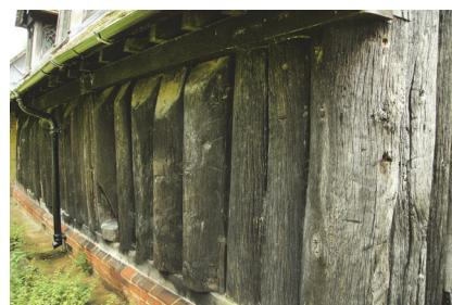
Fig. 2. Greenstead, (England - Essex), a church with wc fragments from 845 - joints of wall beams with a beam of foundations and a crowning beam [6]
